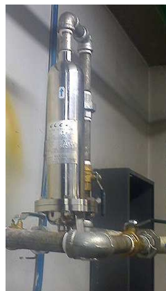
ELCE S-1 Miramar Intercontinental Hotel Panama
